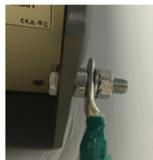
Figure 49 Remote Ground Connection
