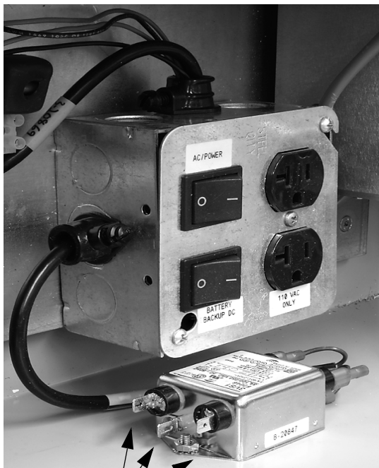
Connect incoming AC line to the input lugs of the AC line filter
